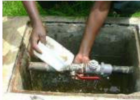
Fig. 5 Testing for gas leakage
