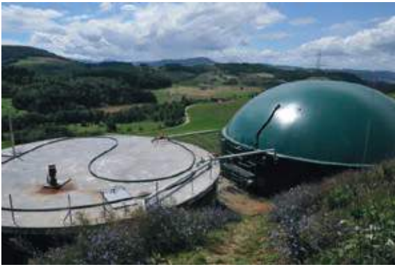
Figure 7.2 View of a mesophilic anaerobic co-digester (left) and an industrial thermophilic anaerobic digester (right).
